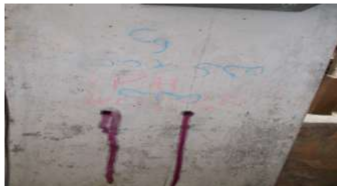
Fig. 4. Depth Of Carbonation Test
